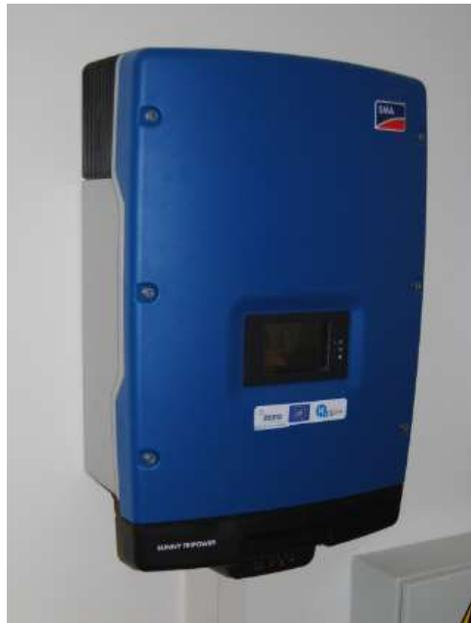
Figura 4. Inversor DC/AC SMA.
